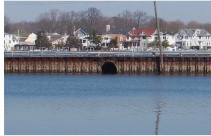
Fisk Avenue Culvert (W-8) over Debbie's Creek and The Glimmer Glass
